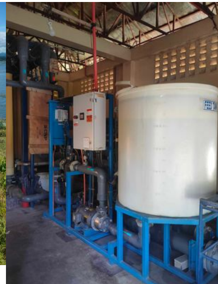
Feed Tank, Circulation Pump and Main Control Panel
