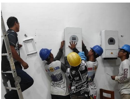
Figure 4. Installation of the Inverters
