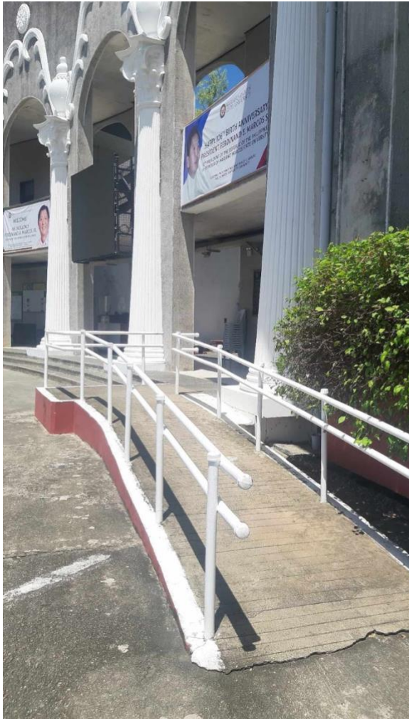
Pedestrian paths for PWDs. All the buildings of MMSU have ramps for PWDs. These ensure their safety as well in getting in and out of the buildings.
