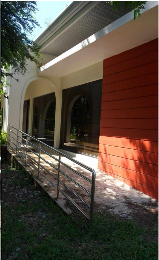
Pedestrian paths for PWDs. All the buildings of MMSU have ramps for PWDs. These ensure their safety as well in getting in and out of the buildings.
