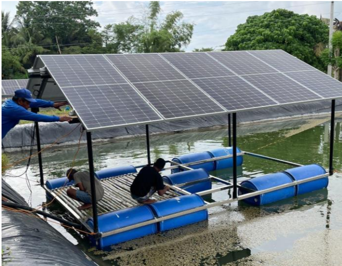
Example of Floatovoltaic Grid tie setup at MMSU Currimao Campus
